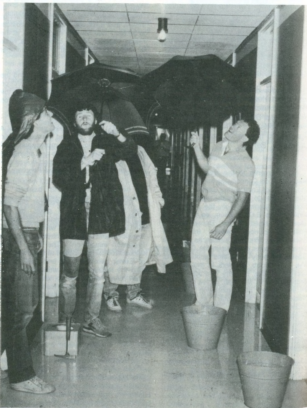
Raising the Roof. Geology Department tribulations while awaiting the arrival overhead of the Economics Department.
