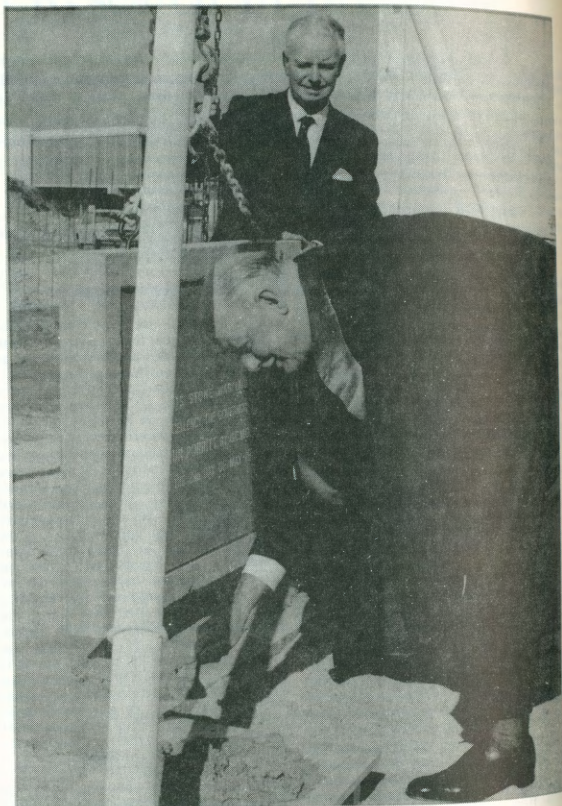
The Governor-General, Sir Arthur Porritt, laying the foundation stone of the James Hight Library at Ilam on Saturday. Behind him is the contractor, Mr C.S. Luney.
