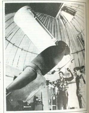
A 24-inch Cassegrain reflector telescope, which has the largest aperture of any telescope in New Zealand, has been installed at the Mount John Observatory, Lake Tekano which is operated jointly by the Universities of Pennsylvania and Canterbury
